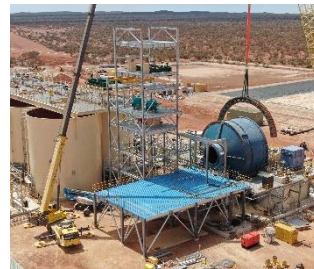
Supply of a 36' x 18' SAG mill – Installation taking place
